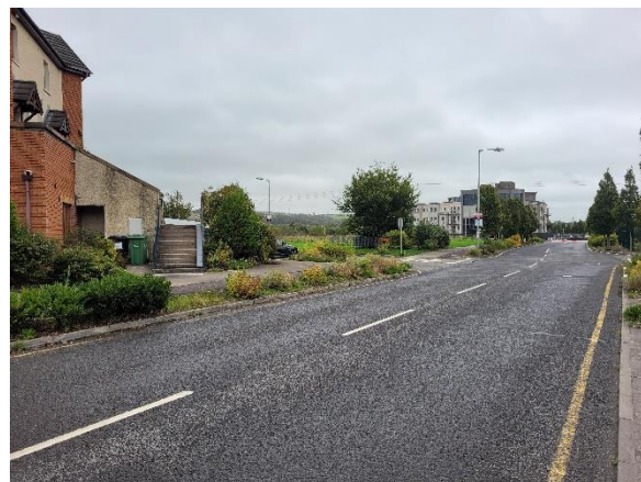
Above right – new access road by Cascade Apartments.
