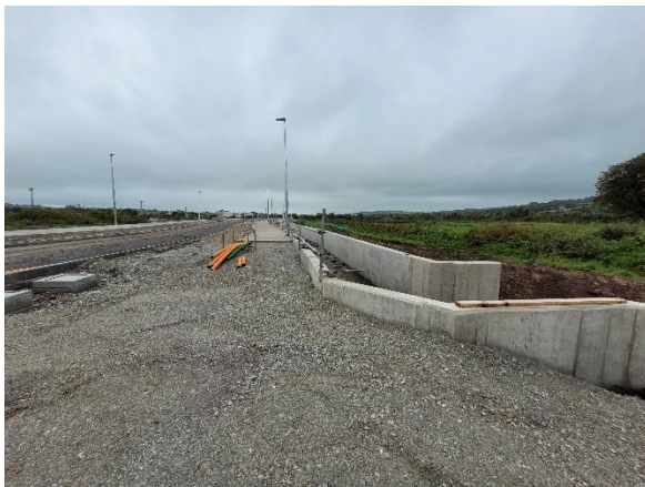
Plate 11-8 Above left – new east west link road
