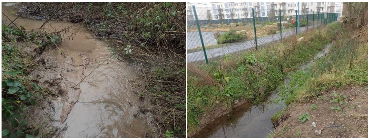
Plate 5.14 Siltation and poor hydromorphological condition implies low ecological value for drainage ditches. Aquatic survey site 3 (left), site 4 (right).
