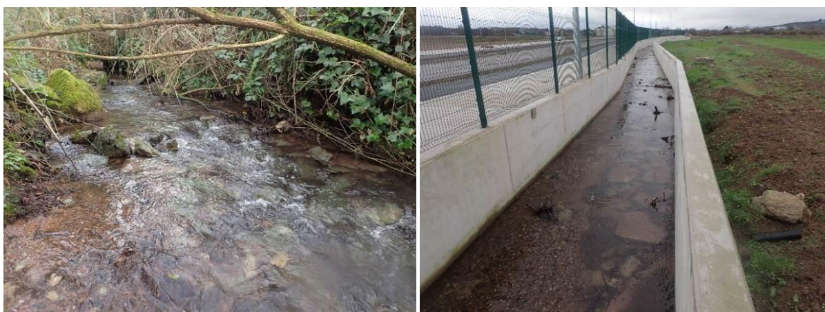
Plate 5.15 Woodstock Stream, an eroding upland river at the eastern boundary of the site (left). A re-sectioned reach of the same waterbody now enclosed by walls and disconnected from its floodplain - drainage ditch.
