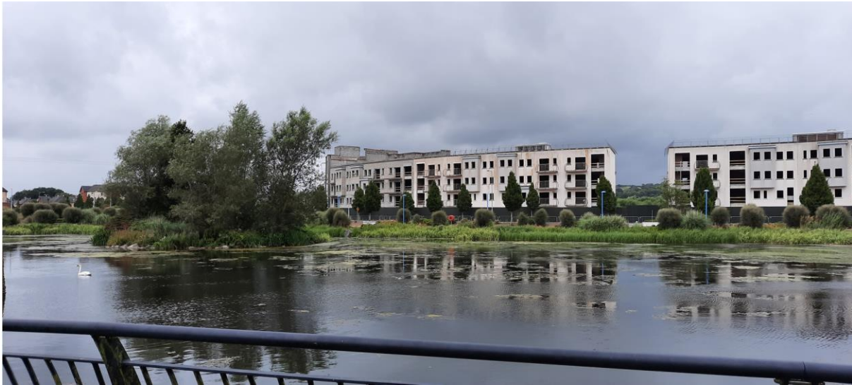
Plate 2-3 Castlelake attenuation pool and adjacent apartments undergoing refurbishment
