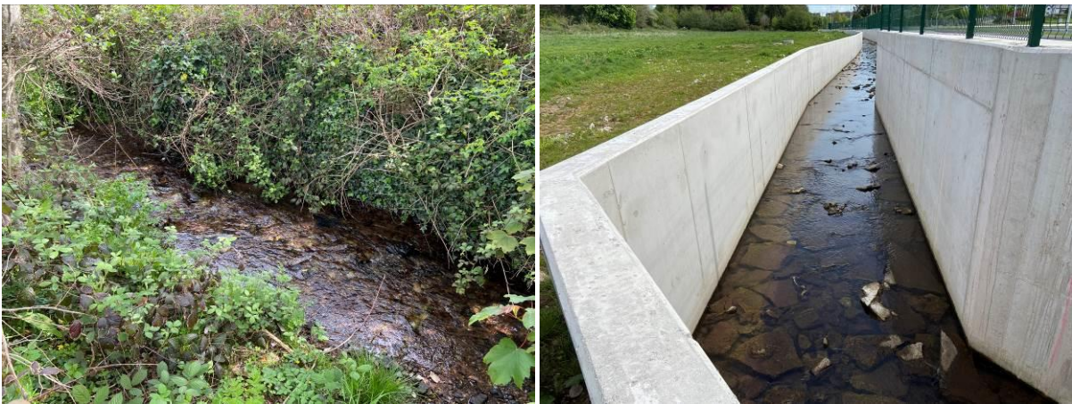
Plate 5.3 Site 4 (left) and Site 5 (right) on the Woodstock Stream.
